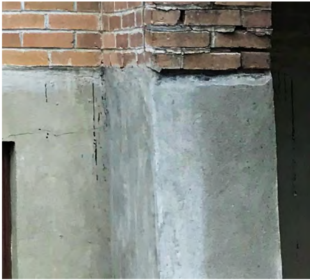
Broken concrete under a failed brick repair on a buttress, a result of water and incompatible mortar stucco
