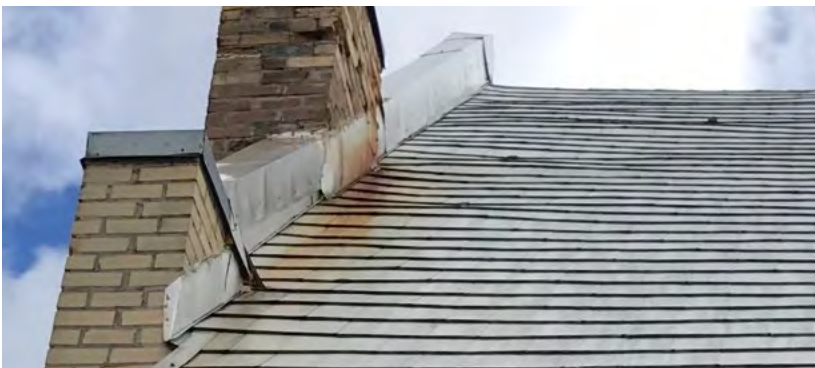
Above: An example of the flashing installation showing the gaps and seams that lead to water penetration of the structure
