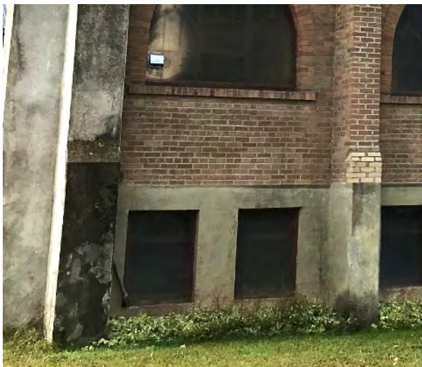
Run off from the roof onto the stuccoed buttresses has caused significant staining
