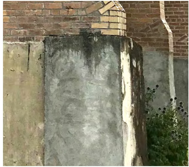
Extensive staining from water on the concrete and a variety of stucco patches on the original foundation
