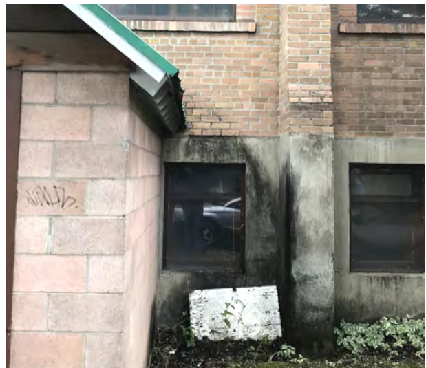
Run off from the roof of the basement fire exit stairs has caused significant staining on the concrete foundation and eroded the mortar of the bricks
